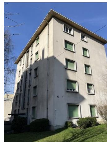
Photo of current building
