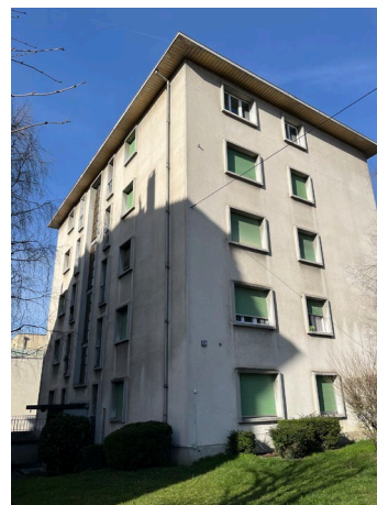
Photo of Current Building
