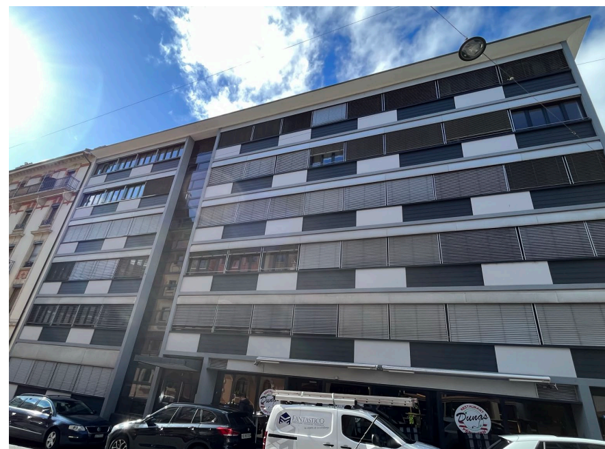
Photo of existing building & attic conversion
